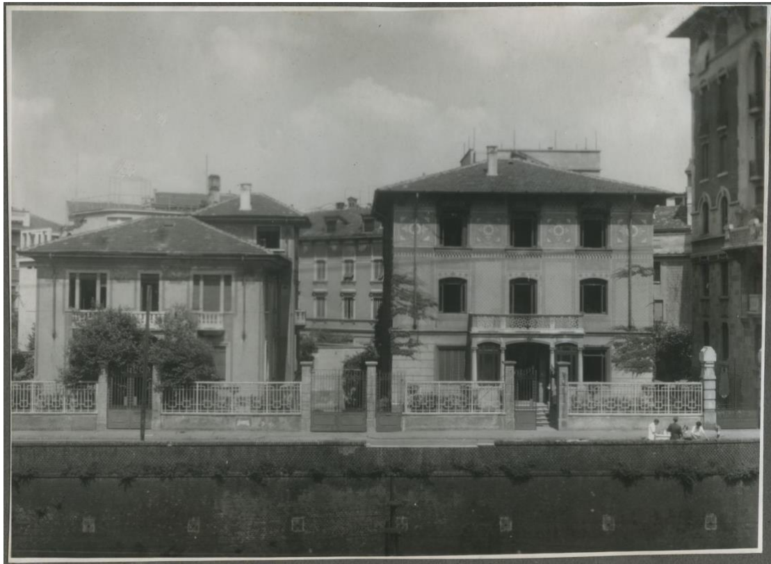
Fig. 1. The two buildings at 6 and 8 via Eupili, Milan. Both buildings housed the Centro di Documentazione Ebraica Contemporanea , 1965-2022., A. D. Schaumann's photographic collection (unprocessed collection). CDEC Foundation Archives.
