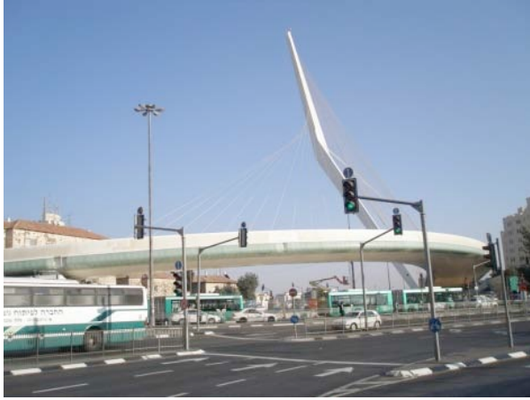
Fig. 2a: The 'Chords Bridge'
