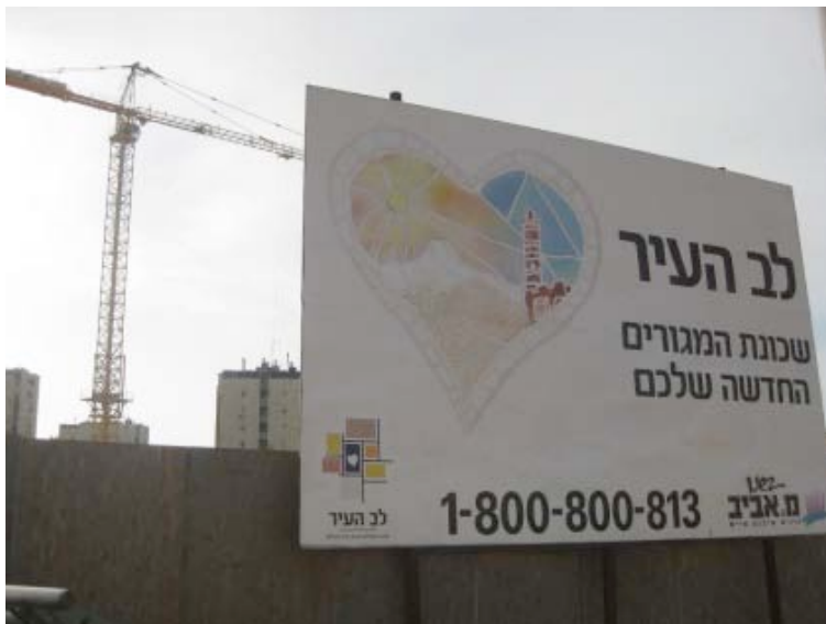
Fig. 3d: Lev ha-Ir neighborhood construction complex
